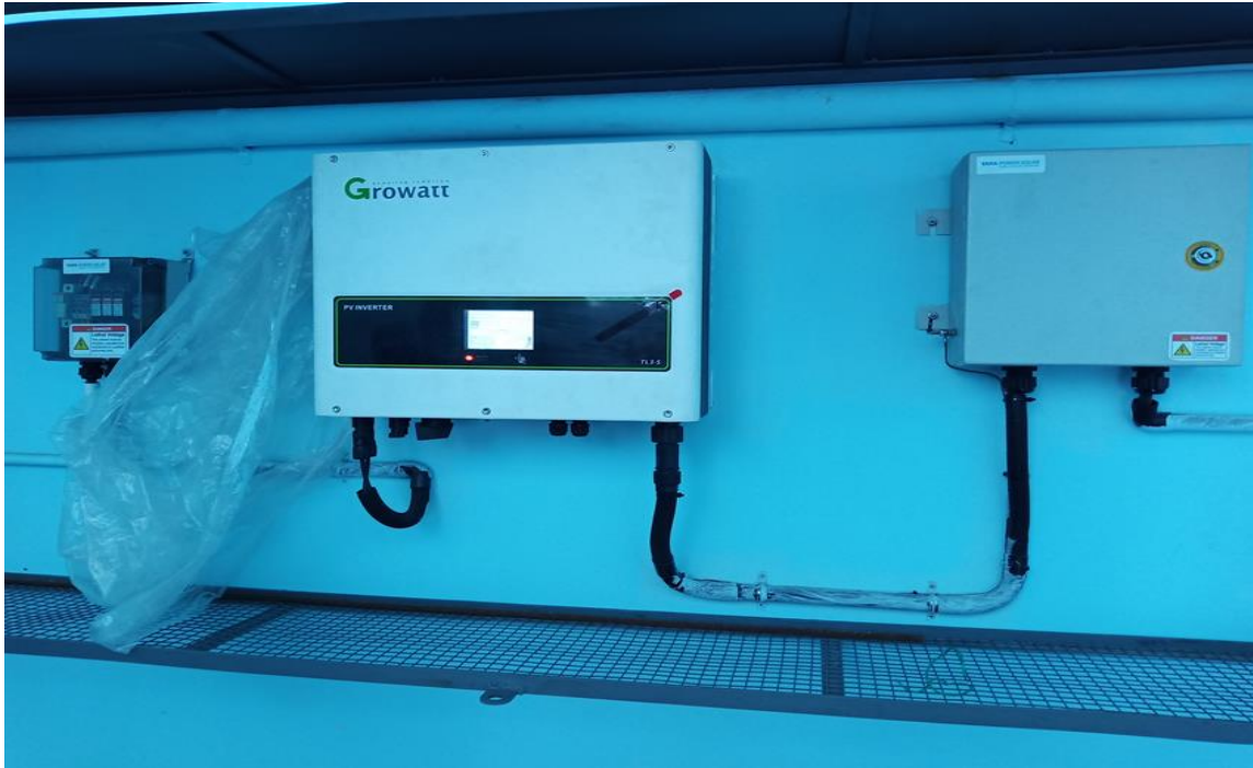
Figure 7.2: Growatt Grid Connect Solar String Three Phase Inverter- 6 KW
