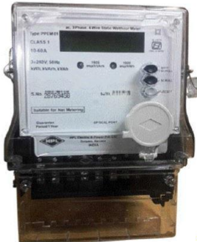
Figure 7.3: Net meter
